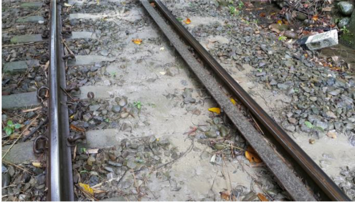
Fig. 2. Pumping photo recorded on 2016.01.05 at Neiwan Branch, Hsinchu, Taiwan
